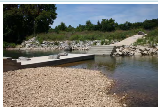
Work on Kelly Slab – Looking Downstream at the Final Product
