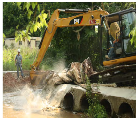
Removing the Slab on Hamstring Creek
