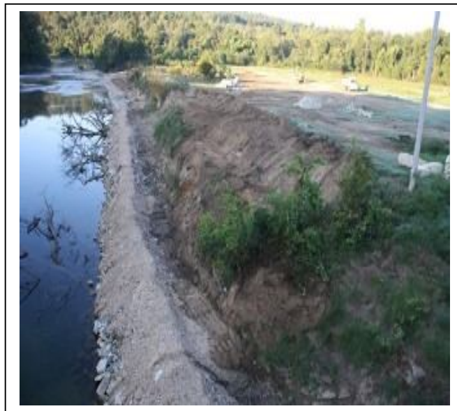
LFSTP Being Built.
