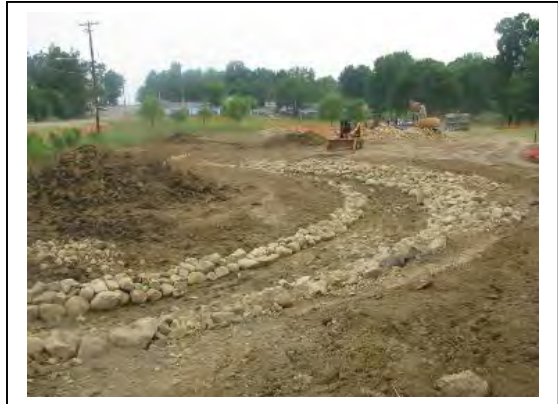
DeQueen Project Mid-Construction
