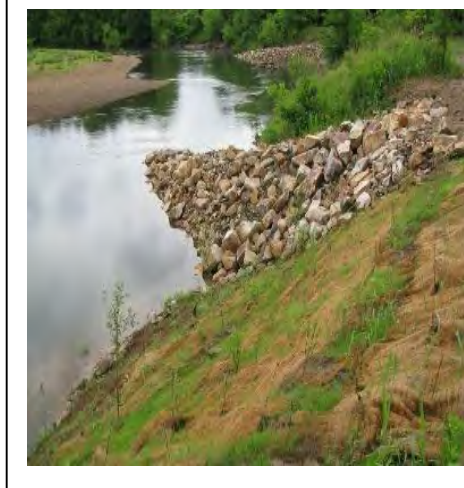
Trees and shrubs planted on the Caddo River to assist in bank stabilization.
