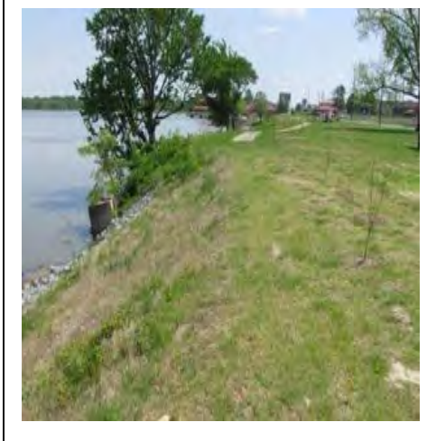
Trees and shrubs planted at Lake Saracen to assist in bank stabilization.
