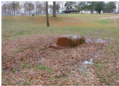
The unsightly artesian well that is to be rehabilitated into an aesthetically pleasing and functioning well system.
