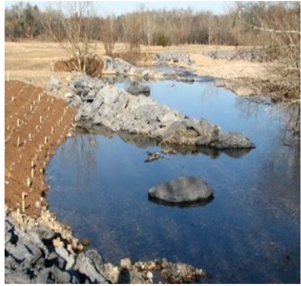
Polk Creek – Completed Project
