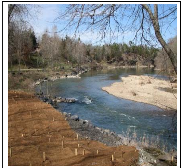
Ouachita River - Completed Project
