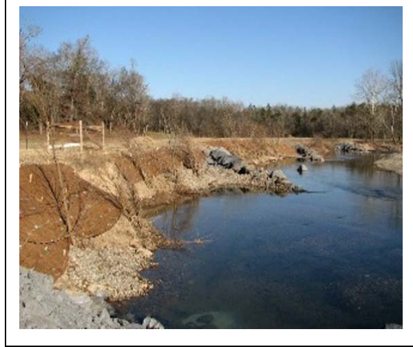
Caddo River - Completed Project
