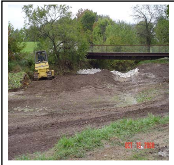
Channel Plug and Upstream Newbury Riffle
