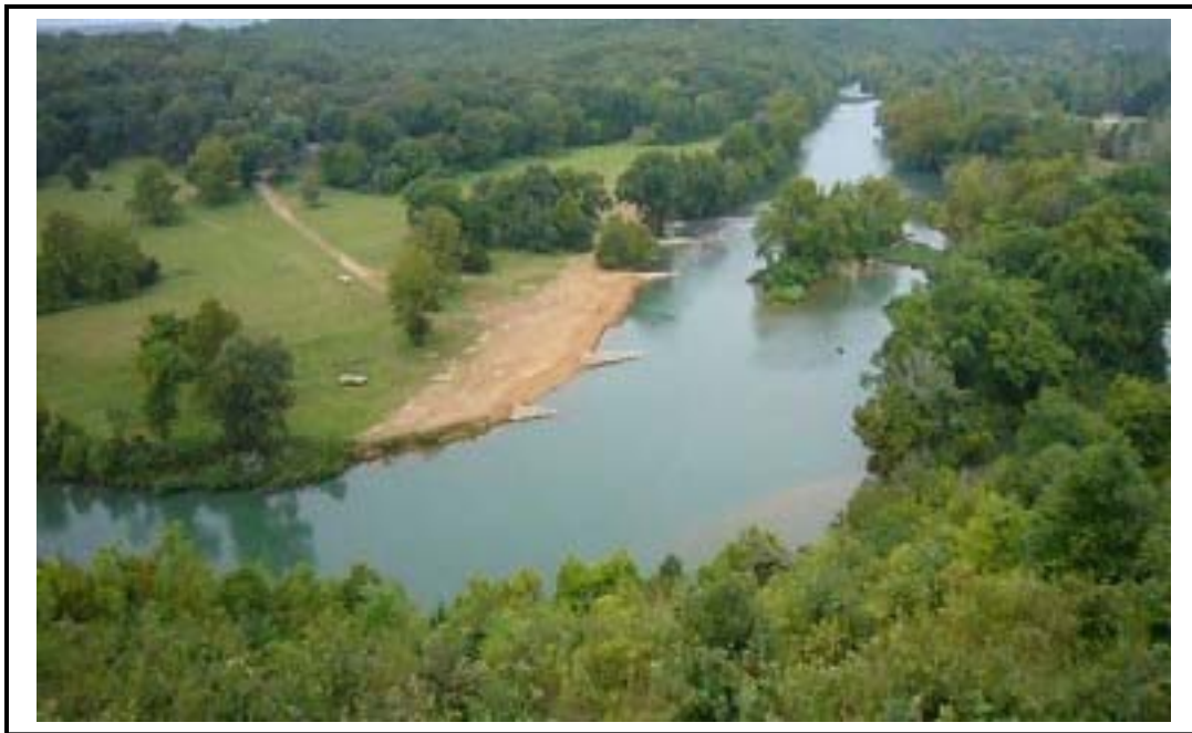
Instream fish habitat improvement and bank stabilization/restoration at work.
