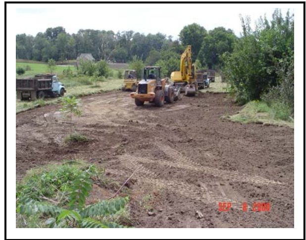
Sod/Top-Soil Removal
