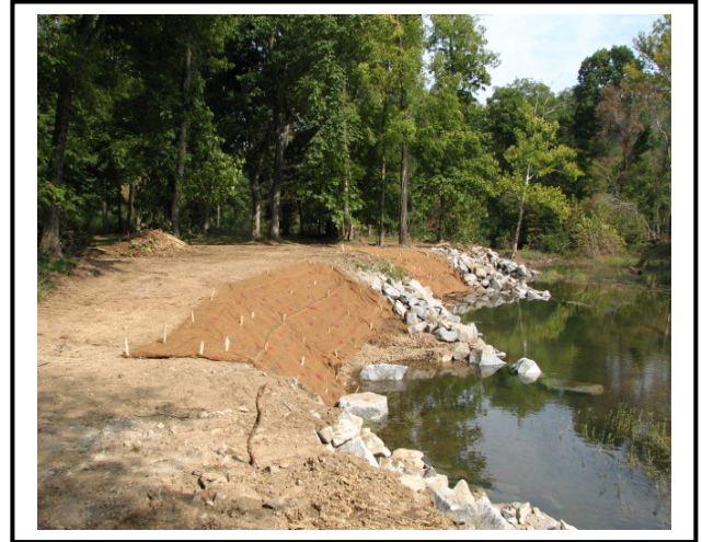
The Installation of Four Rock Vanes and Bank Sloping on the Little Maumelle River
