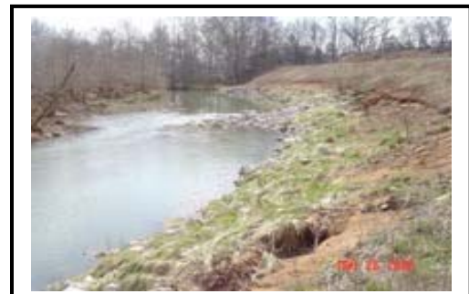
LONGITUDINAL-FILLED STONE-TOE PROTECTION WITH HIGH WATER MARK
